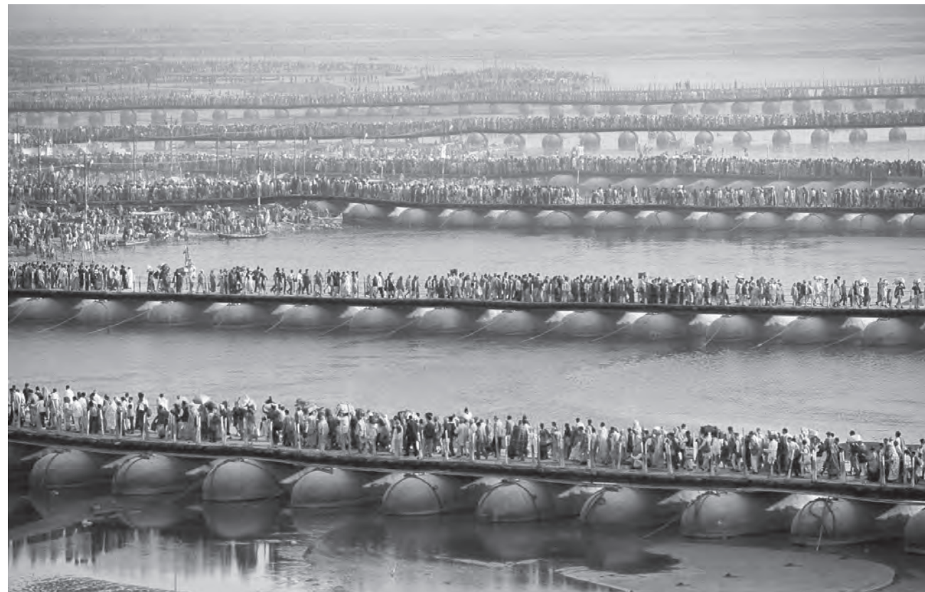
Pontoon bridges at the Kumbha Mela of 2013
