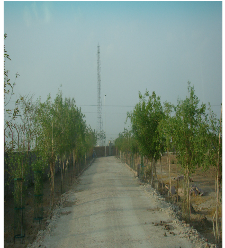
Ring Road alongside the boundary wall now
