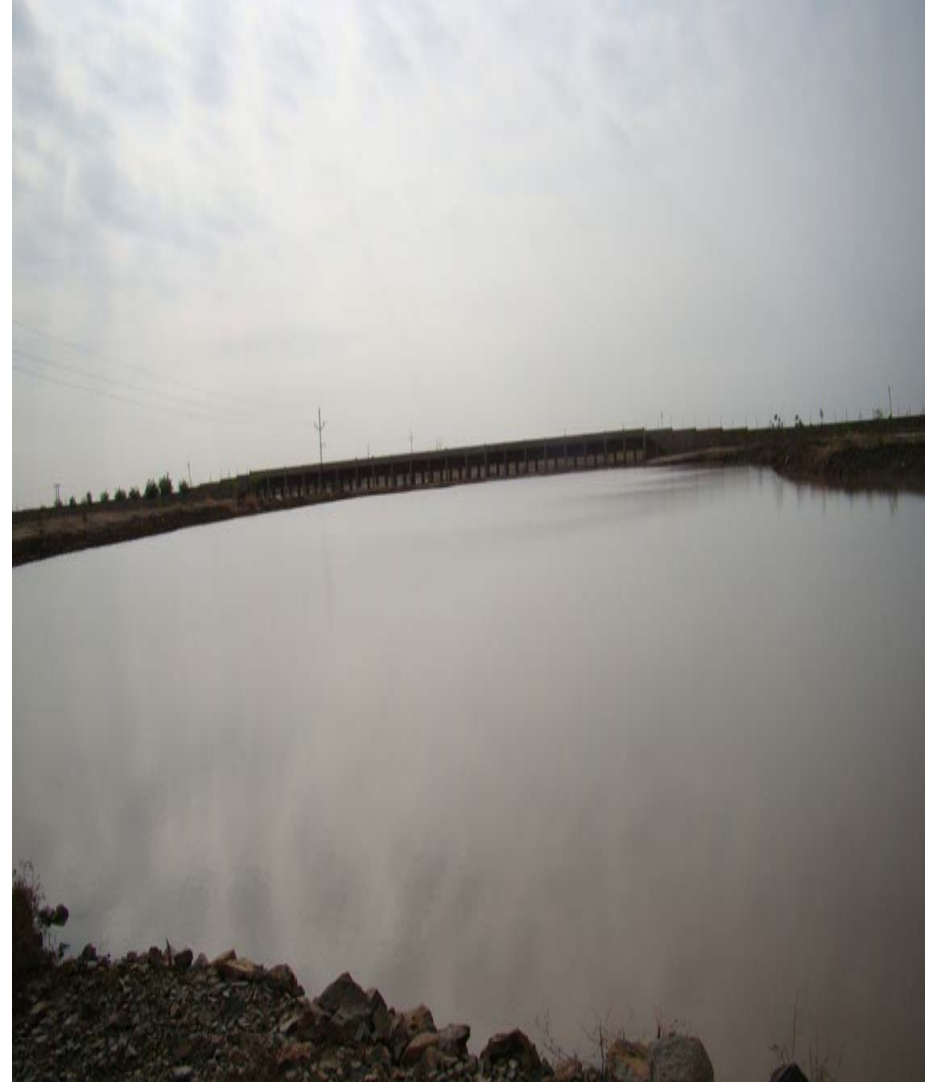
Dugs converted into Lakes
