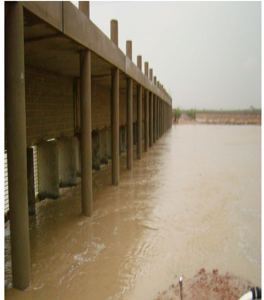
Rain Water flowing in through Bridge
