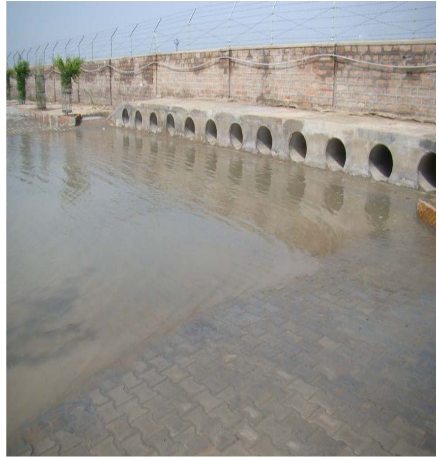
Boundary and Bridges have been constructed Rain water harvesting
