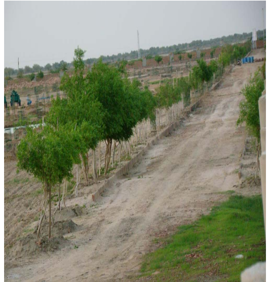
Ring Road alongside the boundary wall now
