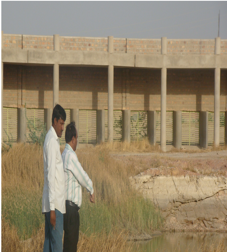
Huge Bridge constructed for inlet
