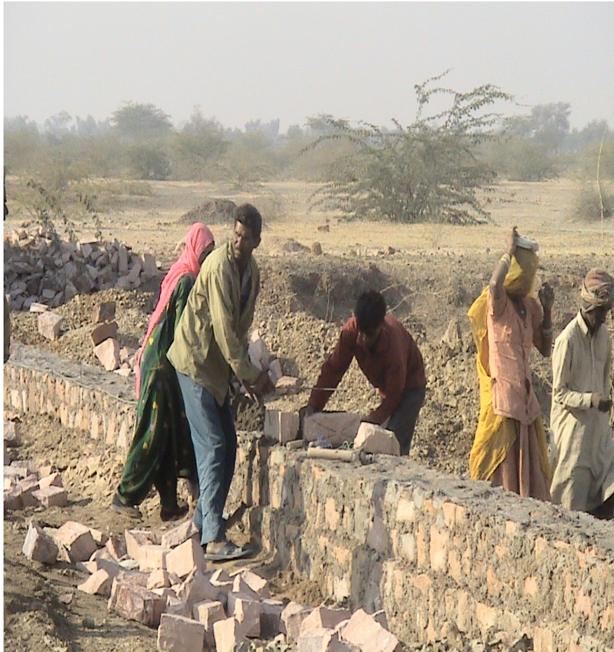
Construction of boundary wall
