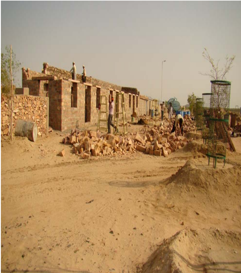
Construction of Project office & Stores with two living rooms
