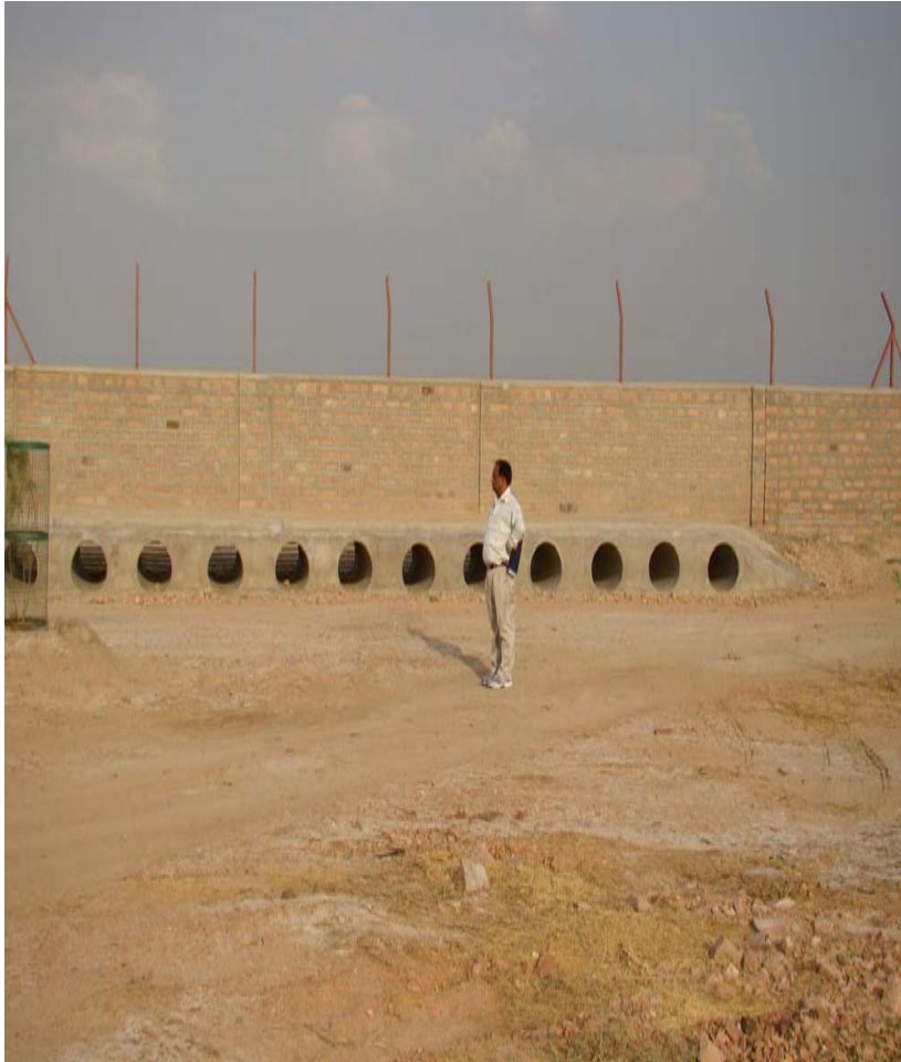
Inlet of Rain Water
